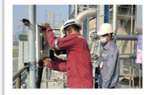
Installation Aquarian 3000 Mini Block#2 HP drum right side
