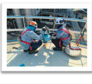
Service annual inspection & calibrate Breather valve w/ Flame arrester
