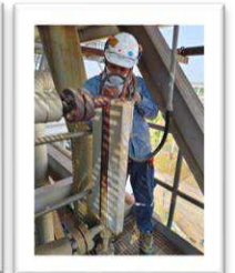
Overhaul sight glass steam drum NPS11 Project
