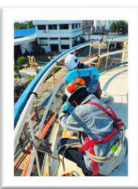
Service annual inspection & calibrate Breather valve w/ Flame arrester
