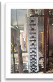
Overhaul sight glass steam drum NPS11 Project
