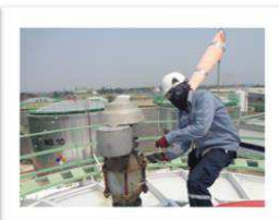
Annual inspection & calibrate Pressure Vacuum Relief Valve at site Project
