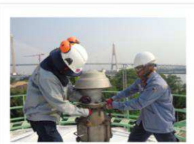
Annual inspection & calibrate Pressure Vacuum Relief Valve at site Project
