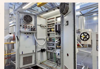
Monitoring and Control cabinet
