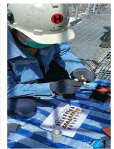
Check and loop test conductivity probe For HP/LP drum (HRSG52) Project
