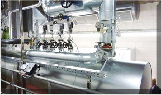
Hot water Boiler
