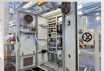
Monitoring and Control cabinet
