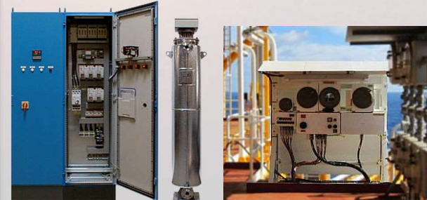
Onshore and Offshore Control Cabinets
