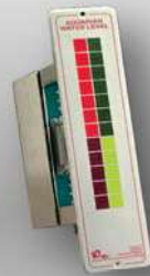
REMOTE DISPLAY (CONTROL ROOM)
